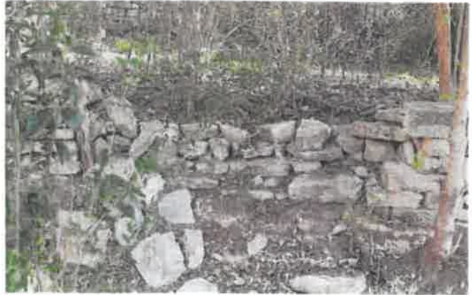
Area of collapse in Section 1B (2018)
