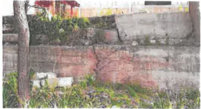
Section 4 is cracked and leaning, and has an overburden of added soil.(2018
