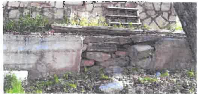
Section 3 is leaning and is cracked. (2018)
